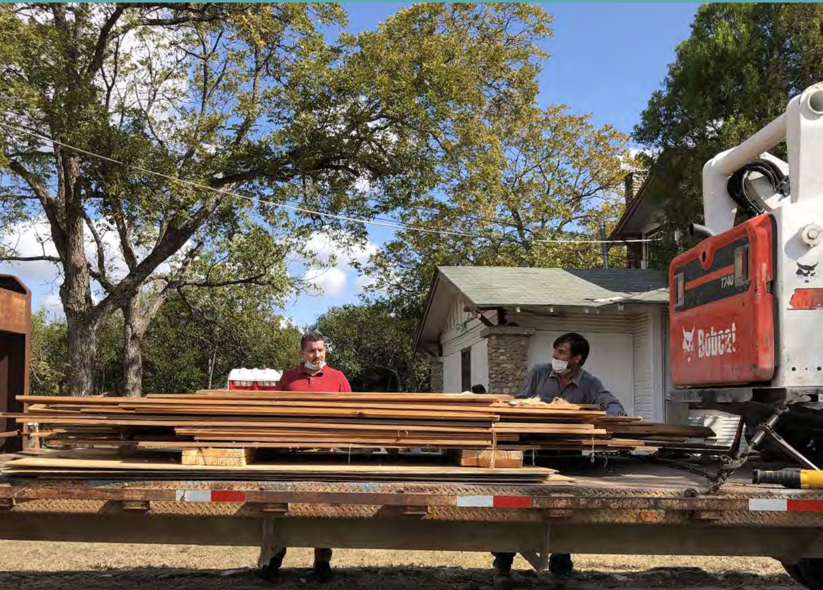
Photo: Participants of City of San Antonio Certified Deconstruction Contractor Training stacking reclaimed flooring and shiplap for transport to off-site warehouse for redistribution. Courtesy Office of Historic Preservation staff.
